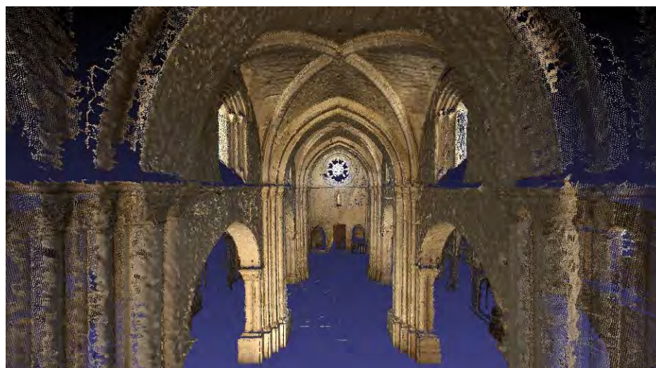
3D digitisation of the Seu Vella cathedral in Lleida, Spain (point cloud of 40 mio points), Visual Dimension
