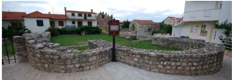
The restored (and partially reconstructed) remains of the Saint John Evangelist church in Biograd
